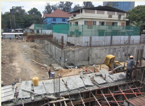
On going construction progress of the Allamano Centre. Let us continue to support this project.
