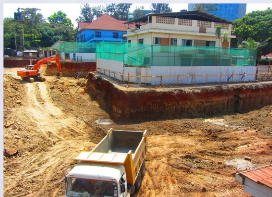
Construction of the Allmano Centre is ongoing, and we can now see the progress of the work. We continue to request prayers and support to help complete construction of this project.
