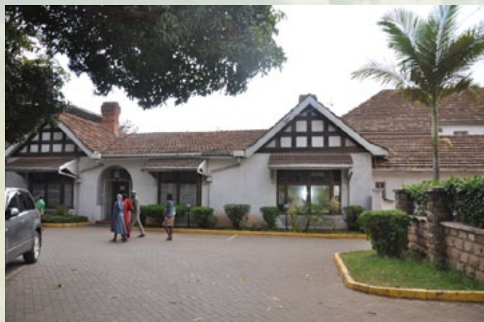
The current office block, which has been in existence since 1950s. It will be demolished to pave way for the new office block. Photo/Anne Gakere
